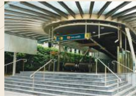
one-north MRT Station
